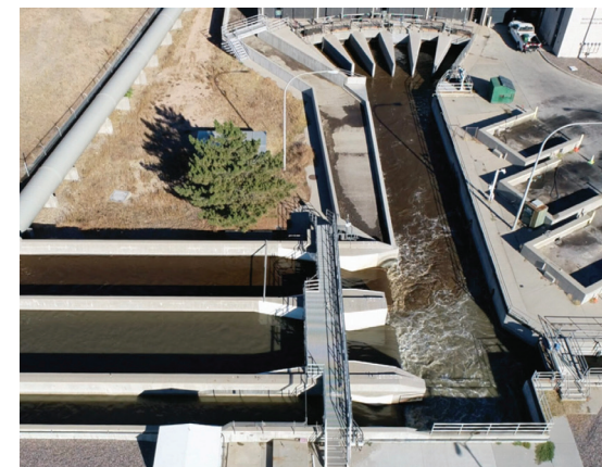
Intake facilities at Metro Water Recovery's treatment plant. The plant provides wastewater treatment for 2.2 million residents, including ECCV customers, in the Denver area.
