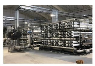
Reverse osmosis filtration units (called "skids") inside the expanded ECCV Northern Water Treatment Plant.
