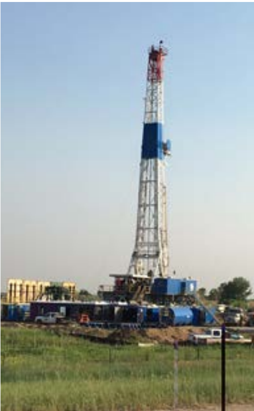
Installation of ECCV Deep Injection Well No. 2, 2016
